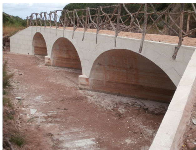
Minorca, Ets Alocs, the discovery of 2013 : One Million of Euros the nice bridge completely useless !
