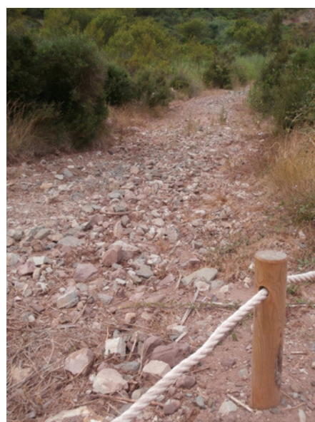
Concrete foundations : 4m wide, 1m deep, very nice facing, ancient track destroyed and access forbidden even for the pedestrians...
